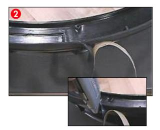
3 Fold the top one-third of the foam rubber tape over and around the top edge of the flashing.
